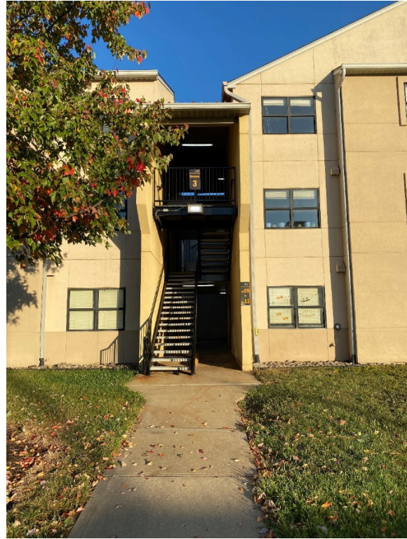
Norse Hall, New Stairs and Landings
