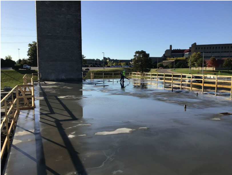
Finishing Concrete, 2 nd Floor New Residence Hall, September 29, 2020
