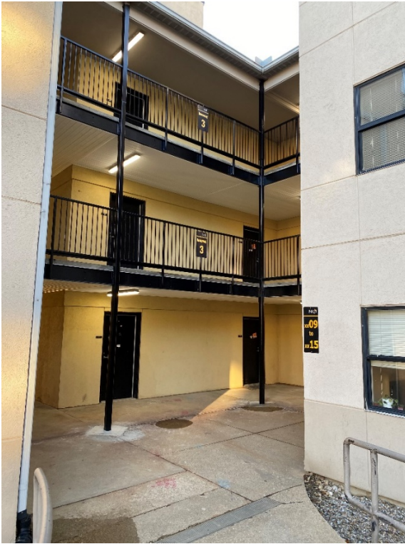
Norse Hall Exterior Repairs
