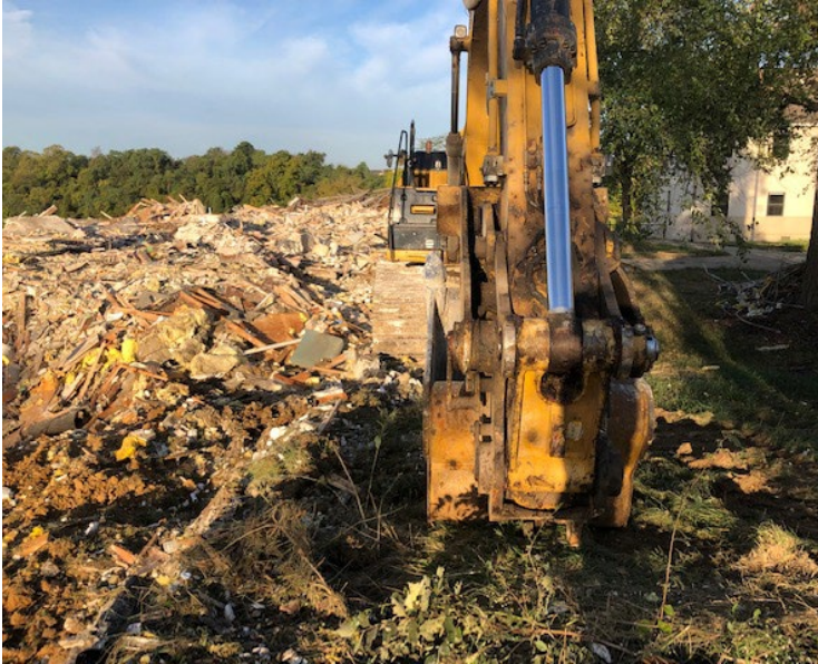
Demolition of Oak Hall, October 1, 2021
