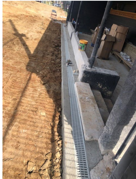
New Trench Drain along Field Edge
