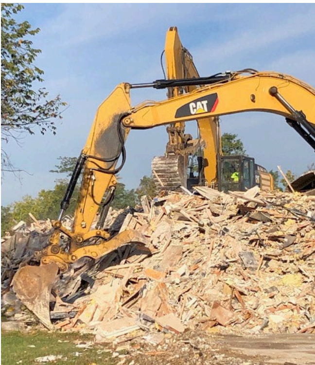
Demolition of Oak Hall, October 1, 2021
