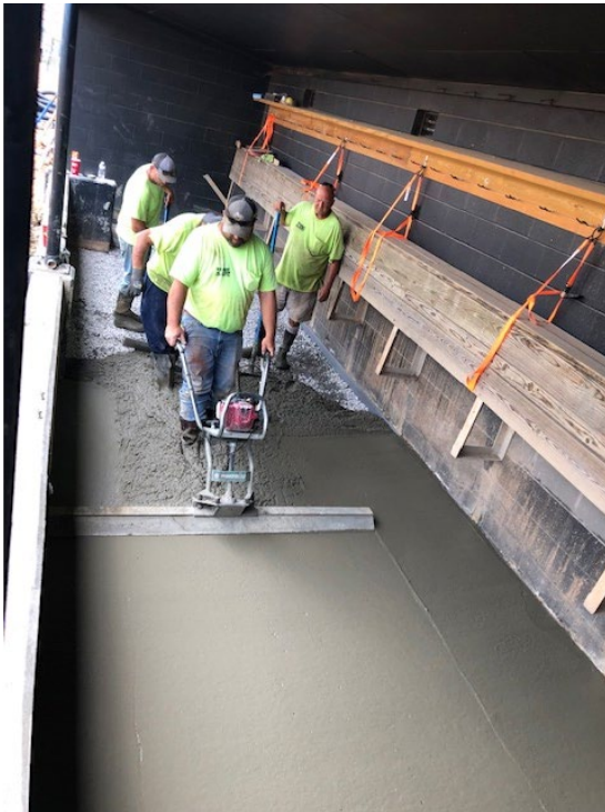
Structural Repairs Complete, with New Floor
