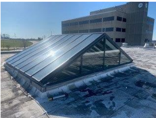
One of two existing skylights that will be replaced.
