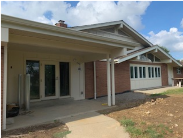
University Police Front Façade
