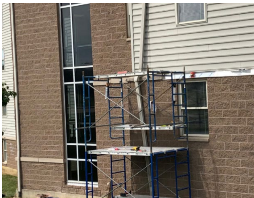
Façade Repairs Underway at University Suites
