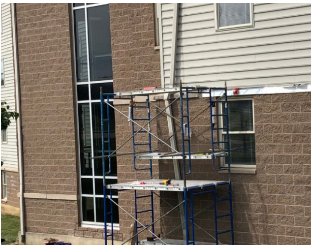
Façade Repairs Underway at University Suites
