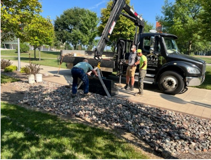
Granite Monument being installed in August
