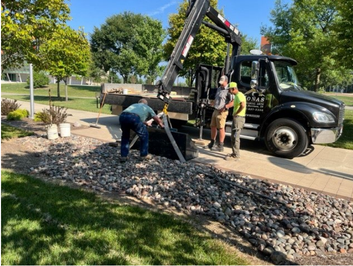
Granite Monument being installed in August
