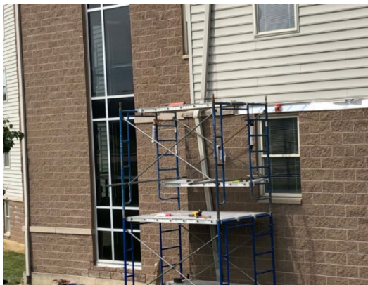
Façade Repairs Underway at University Suites
