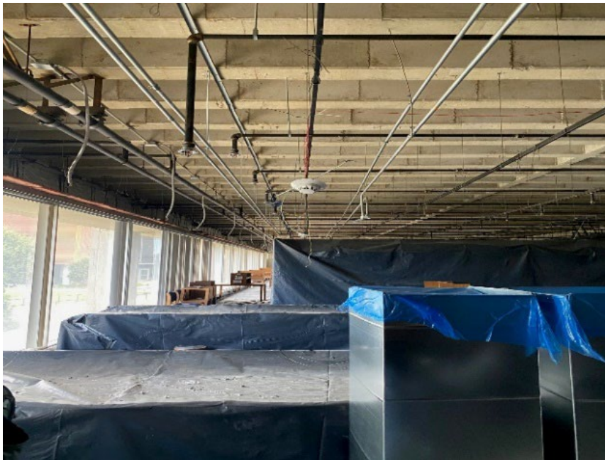
Demolition of HVAC is Complete in the Nunn 2 nd Floor Library
