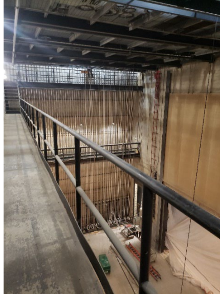
Corbett Theatre Fly System being replaced (photo taken from Corbett stage and from 4 th floor catwalk above Corbett stage). Early October 2024.
