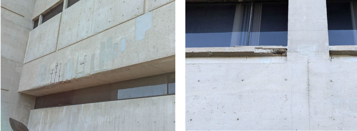
Repairs, patching and cleaning underway on Nunn Hall
