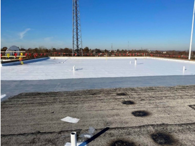
Campbell Hall Roof Restoration Underway
