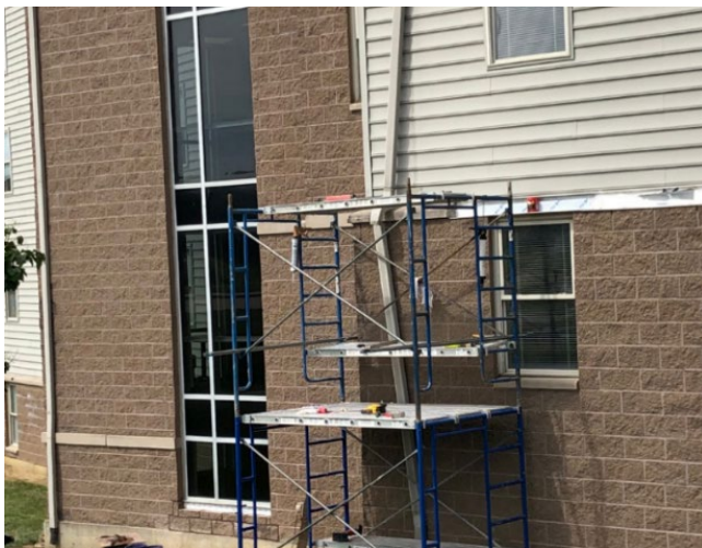
Façade Repairs Underway at University Suites
