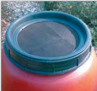
A window screen placed over the barrel opening (left) or a gutter strainer placed in the downspout opening (right) will keep leaves and other debris out of the rain barrel.
