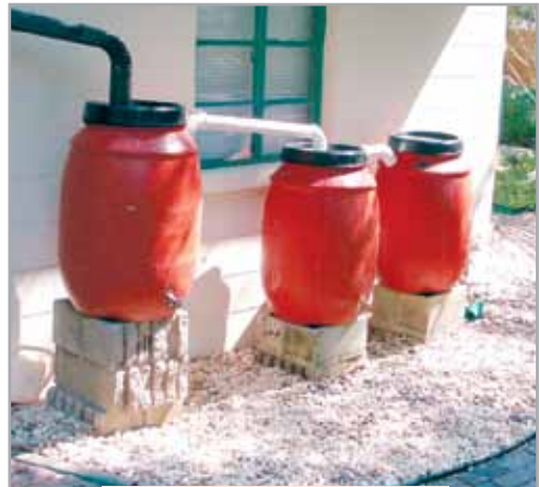
Multiple barrels provide for greater water storage.
