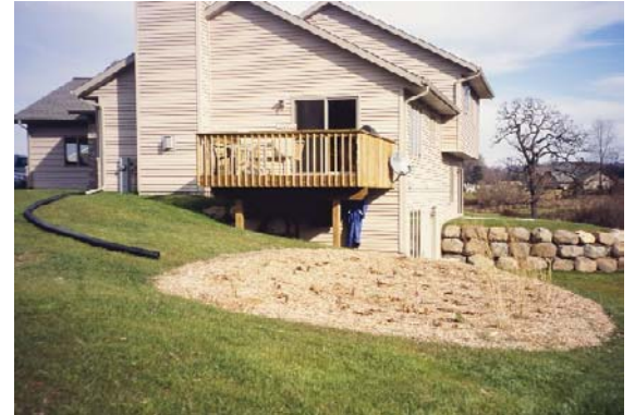
An extension of PVC pipe helps direct downspout water to this rain garden.
